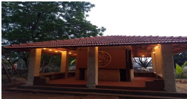
Low cost rammed earth building for coffee center
