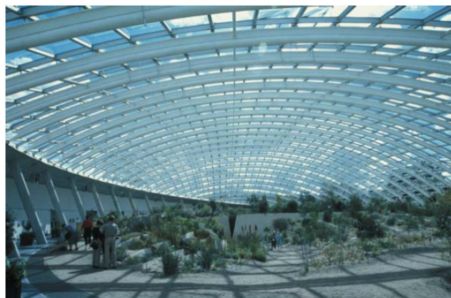
Figure 9.2 The Great Glasshouse, Carmarthenshire, Wales, Foster and Partners, 1998. Arched roof.
